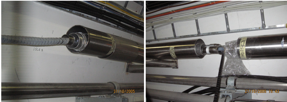
FIGURE 6. Cable bundle insertion in type-1 DSL (left), and extraction at a branch (right).
