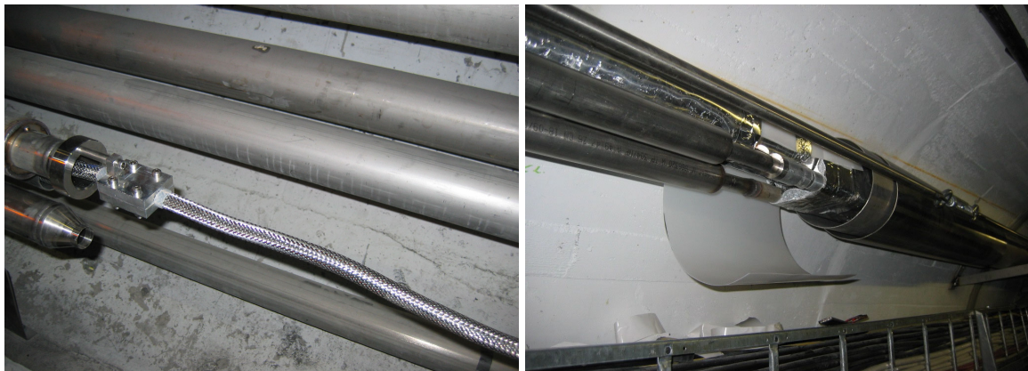
FIGURE 7. Type-2 DSL view of cable with wavy over-length pattern and clamp (left), general view of DSL at thermal compensation location (right)
